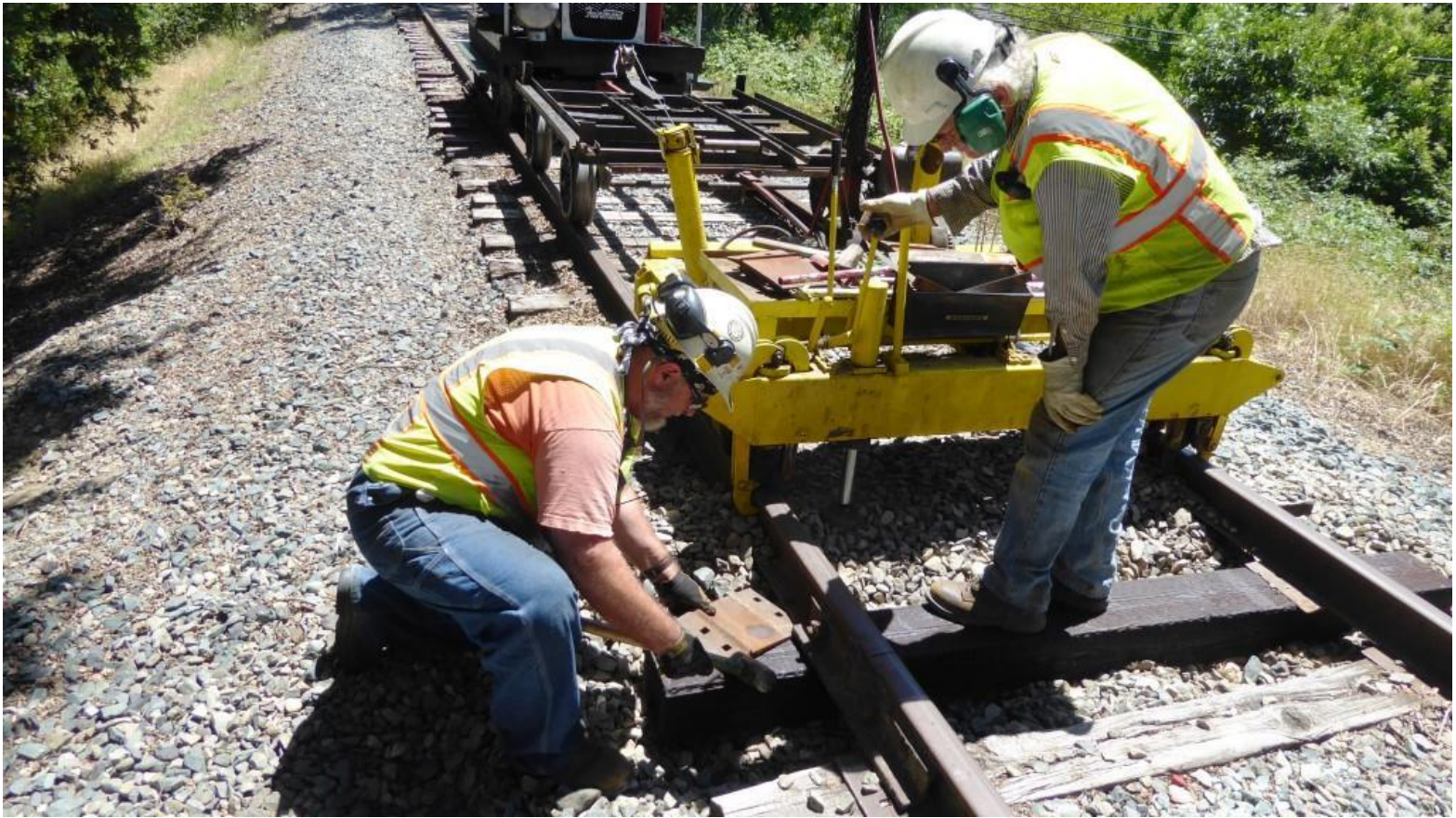
After lunch, Mike F. and Steve plated the ties under joints with special joint-plates
