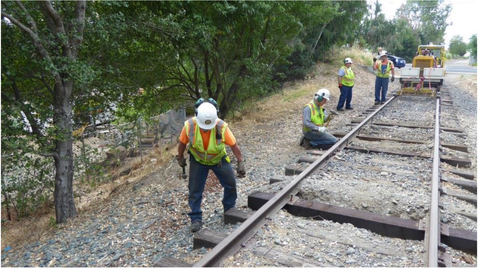
At Mile Post 3.52 (Sutterville Road), Joe and Steve, set spikes into new ties
