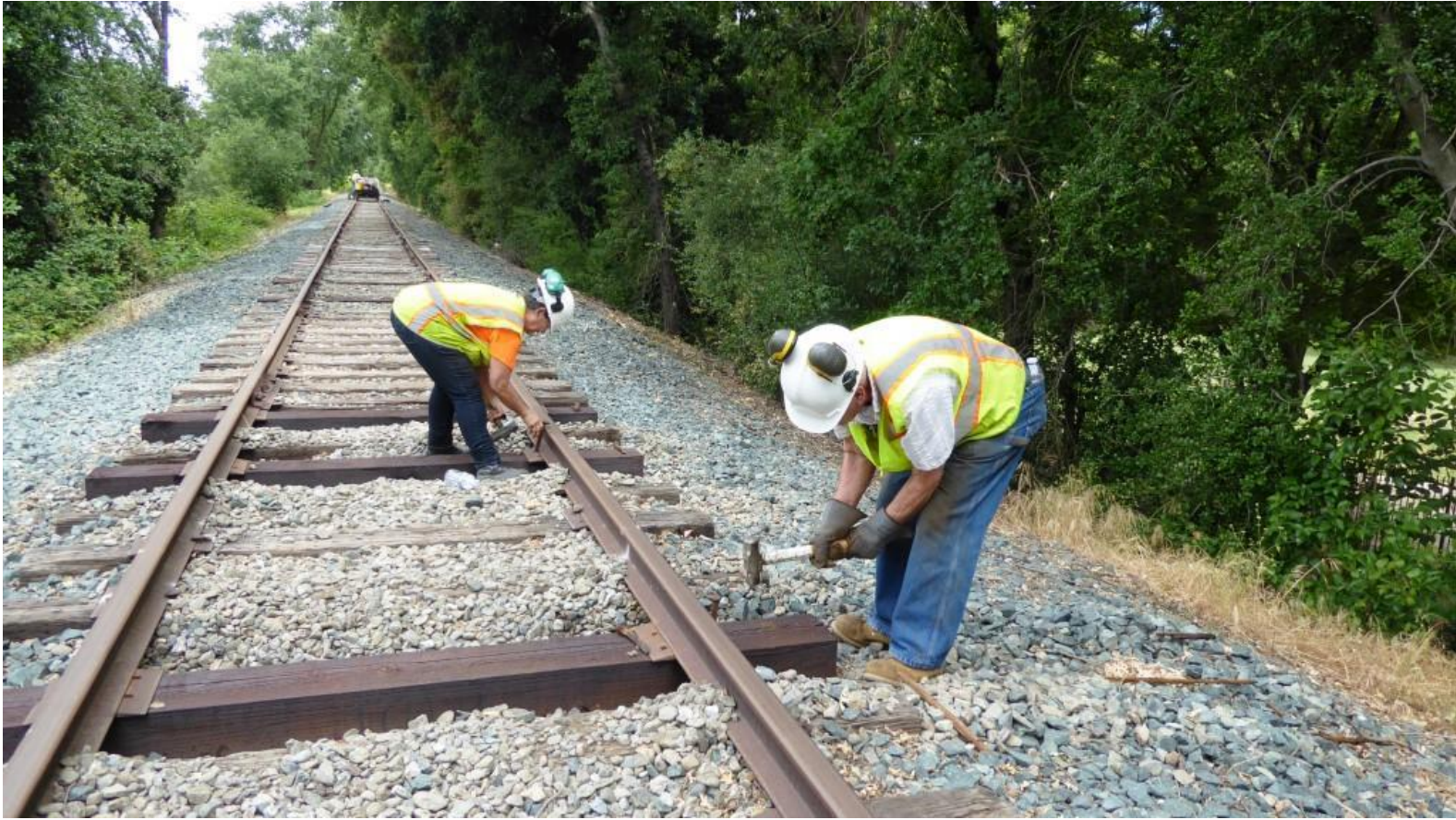
Pam and Clem work their way up the line setting spikes
