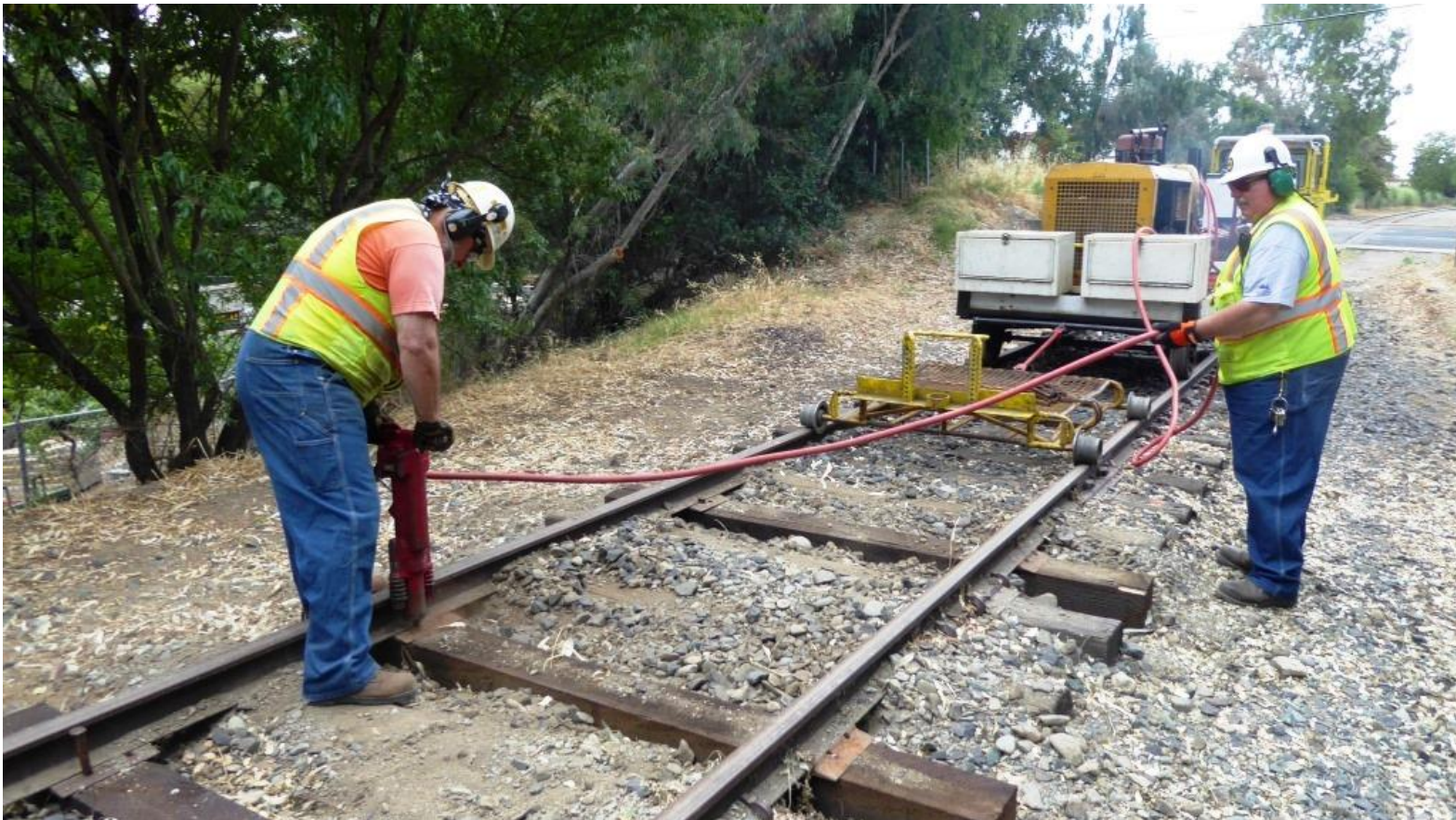
Mike F. drives spikes with the pneumatic spike-driver and Harry manages the air-hose as Alan follows slowly behind shoving the compressor
