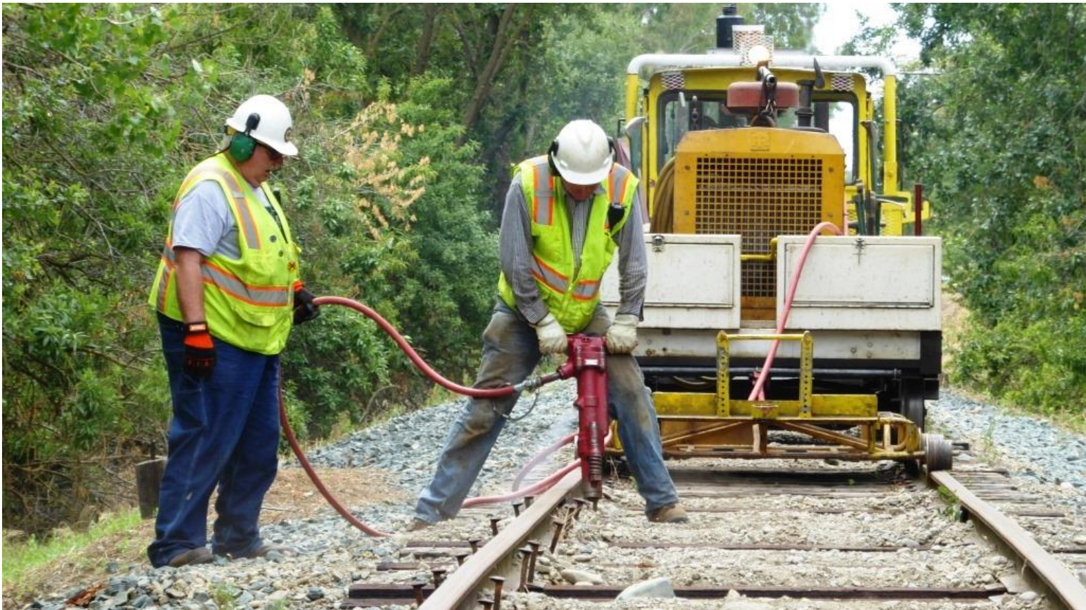
Harry, Steve, and Alan follow behind driving the set spikes with the pneumatic spike driver
