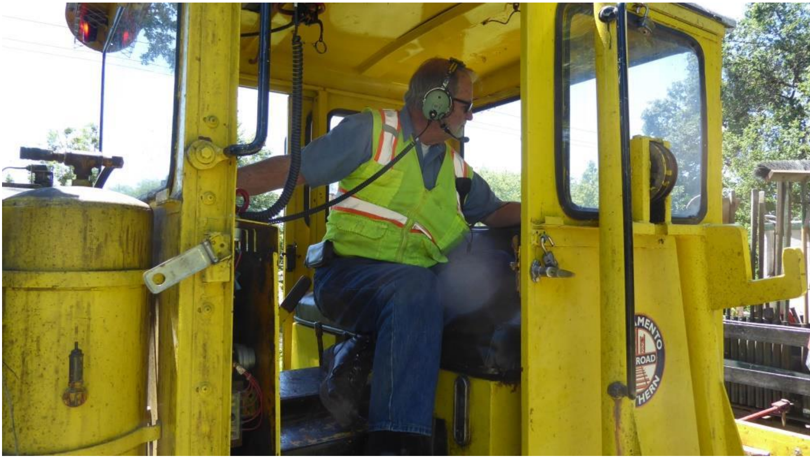
Alan at the controls of the Kalamazoo keenly follows the signals of the spiking crew as he slowly shoves the compressor up the line
