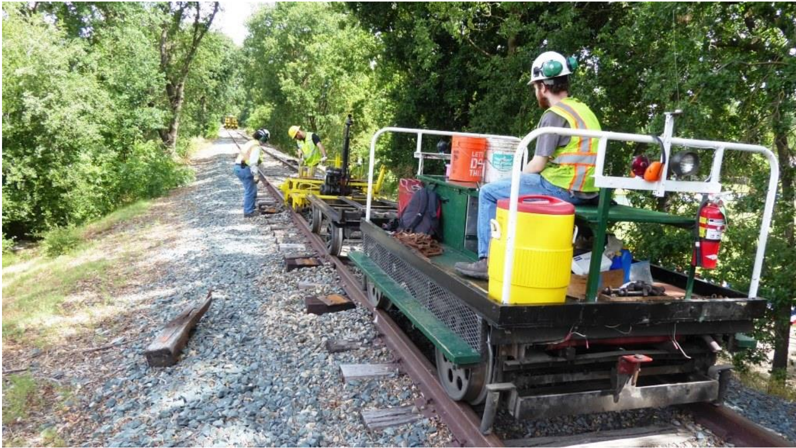
Matt on the motorcar provided head-end power for positioning the rail-lifter
