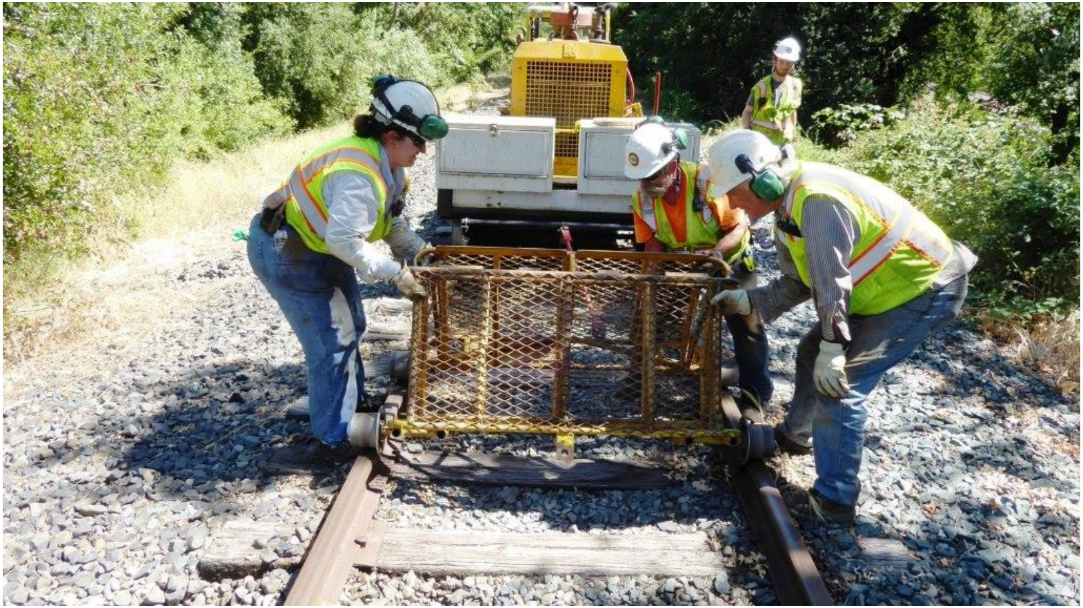
Heather, Joe, and Steve take apart the Nolan Track Cart to stow with the compressor
