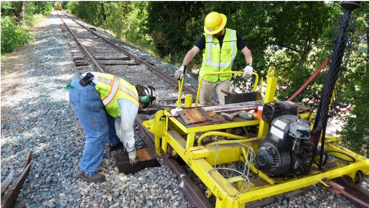
Chris operates the rail-lifter as Heather places a tie-plate
