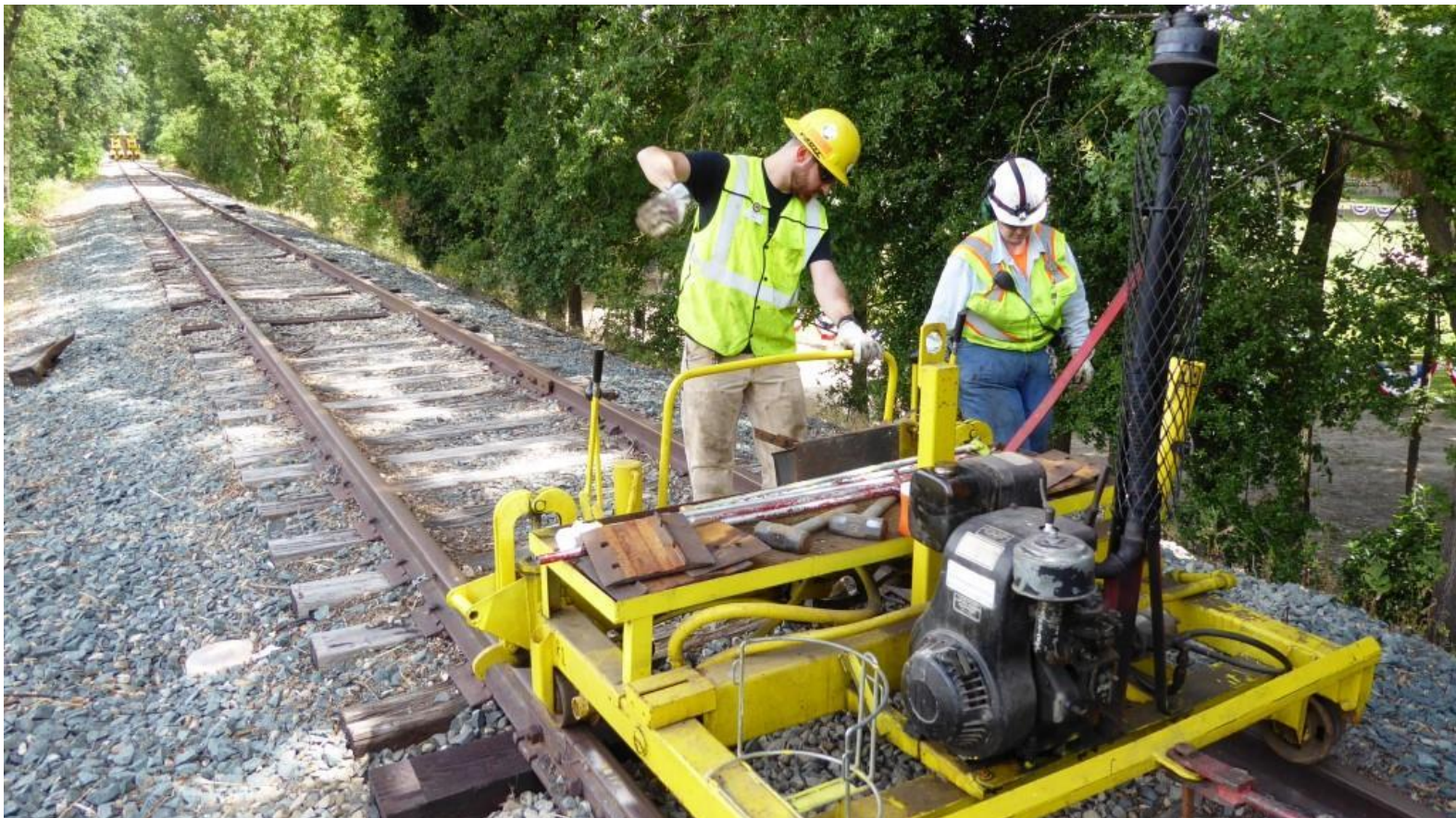
With the lifter over the next tie to be plated, Chris signals Matt on the motorcar to stop
