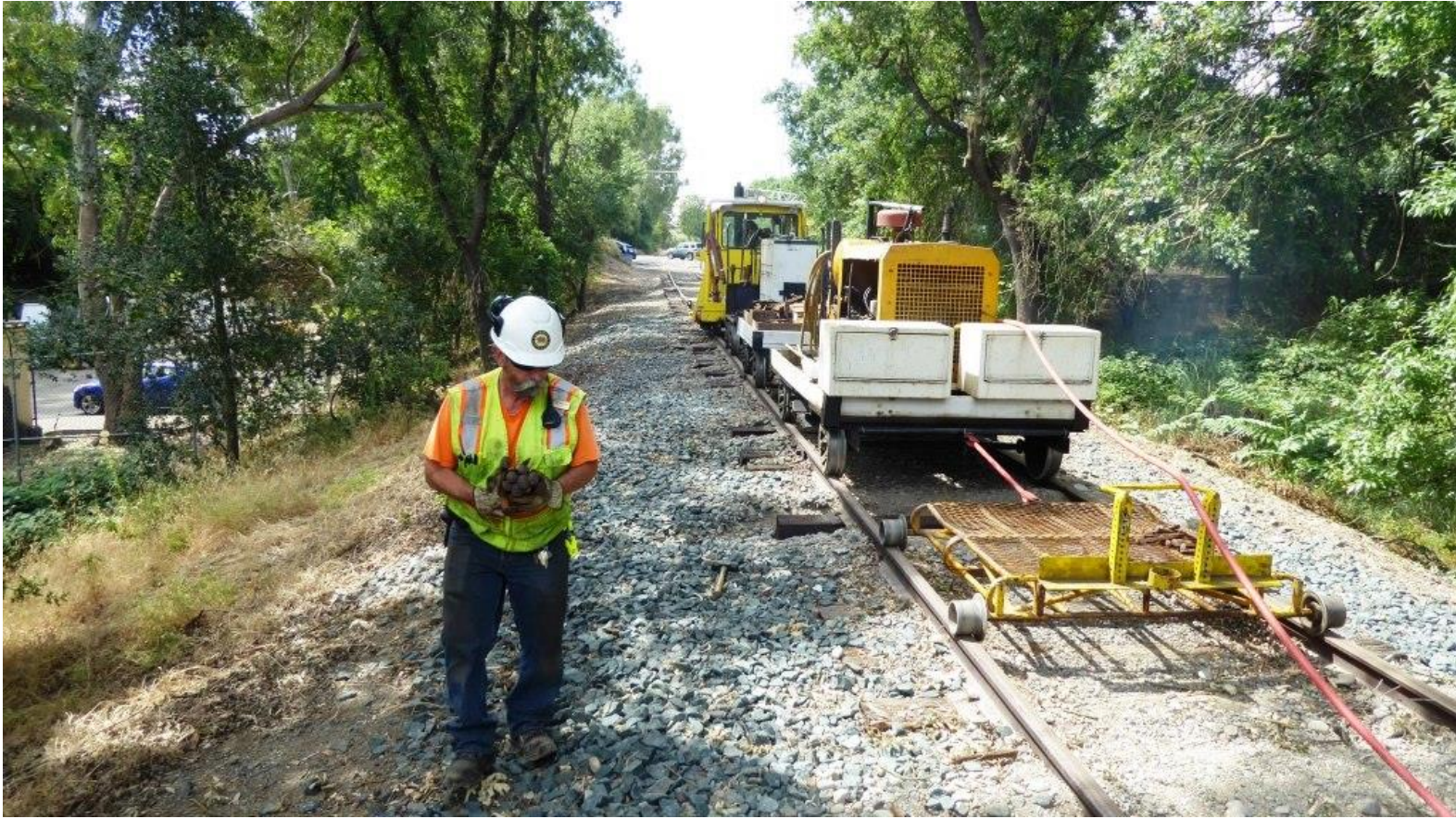
Joe distributes fresh spikes at each new tie
