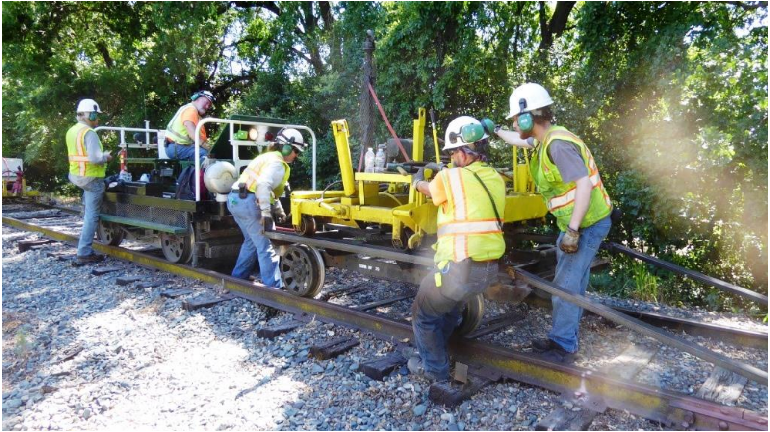
Heather, Joe, and Matt load the rail-lifter onto its carriage
