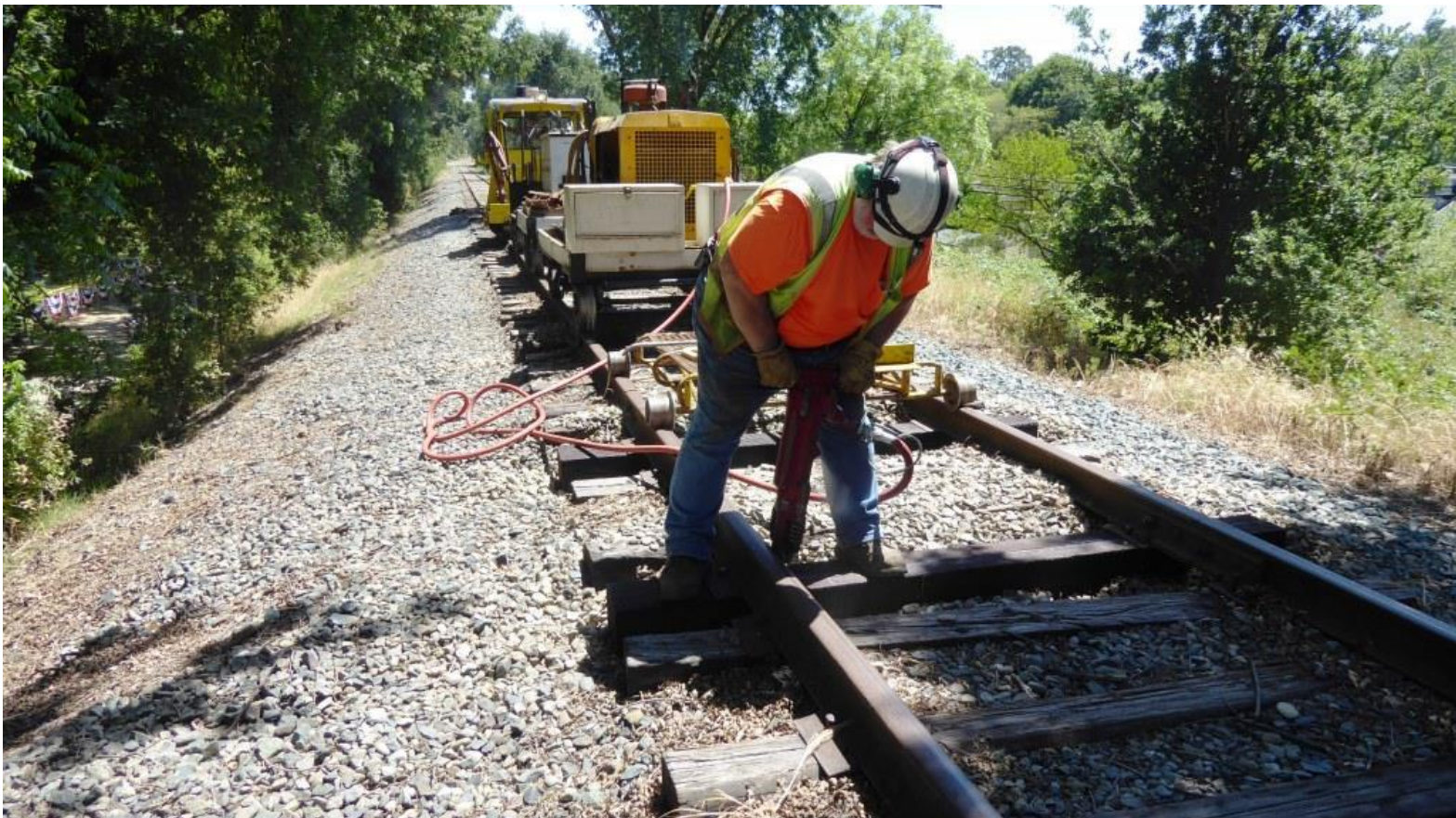
Frank took up the pneumatic spike-driver to drive some spikes.
